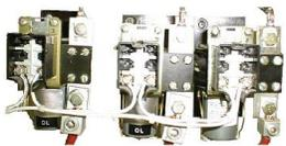
Overload devices must not have loose connections or evidence of overheating
