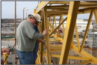
Routine inspections play an essential part in establishing and maintaining the quality of Weight Handling Equipment maintenance, and, are divided into three areas:
